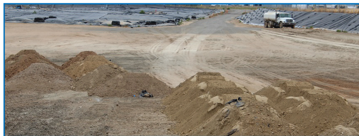
The Consolidation Unit accepting excavated soil from 2019 field season activity. The CU will be closed and covered for the winter.
